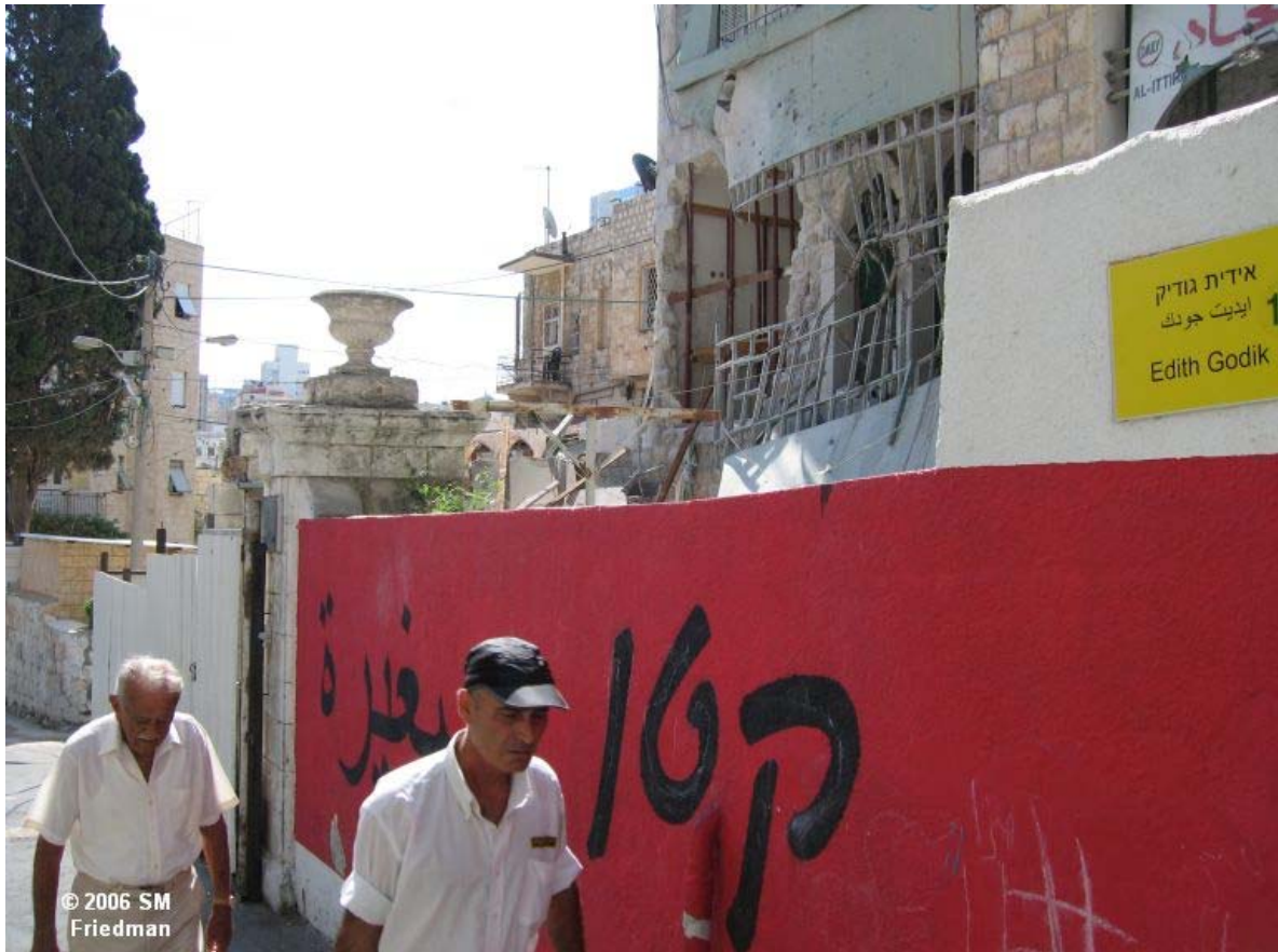
Katyusha missile damage on residential building , Arab neighborhood, Haifa, Israel.
